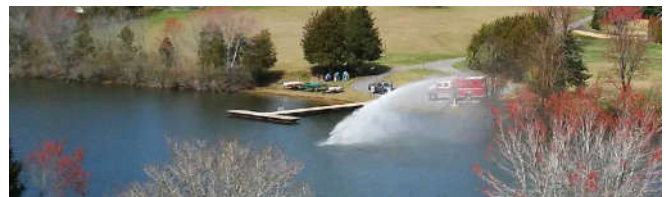
Fire Department test of dry hydrant at the lake
