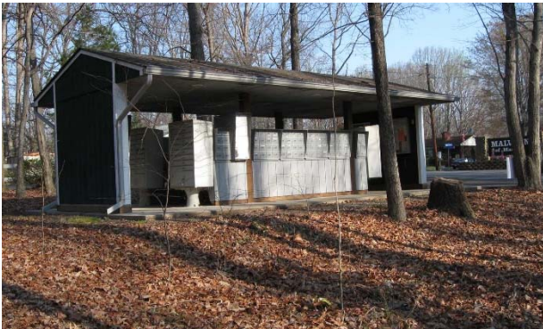
Siding, roofing, painting, cleaning
