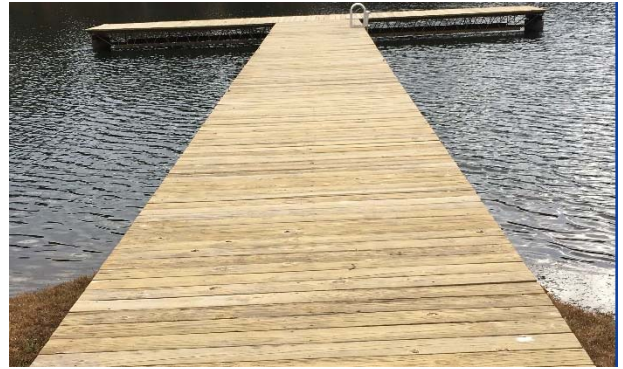
Resurfacing, staining our dock
