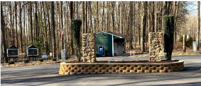
Entrance island work-in-progress
